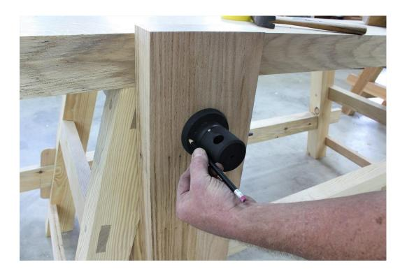
Mark the screw locations at the hub flange and the nut. Remove the vise screw and bore pilot holes for the screws.
